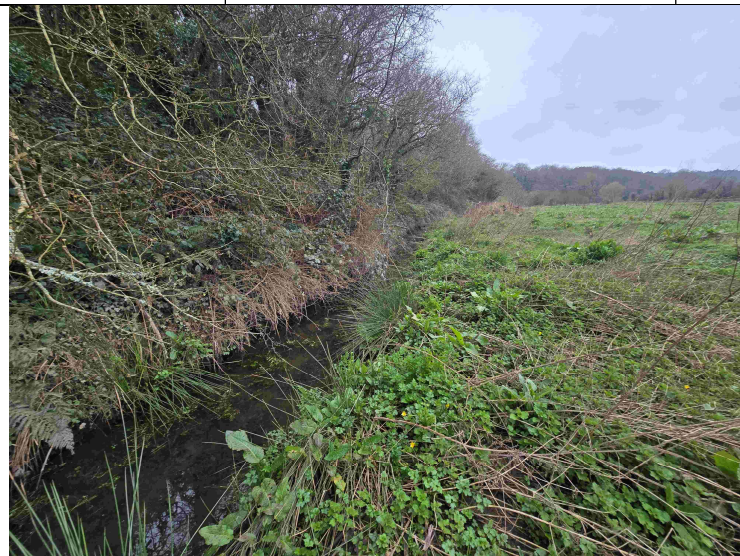
P14. Millrace southwards
